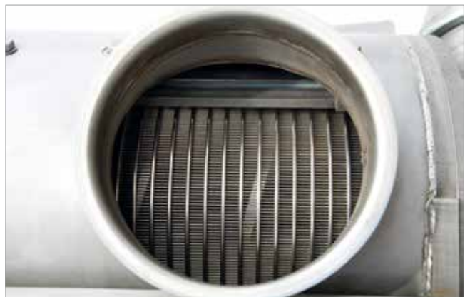
Inspection opening in the screen housing
